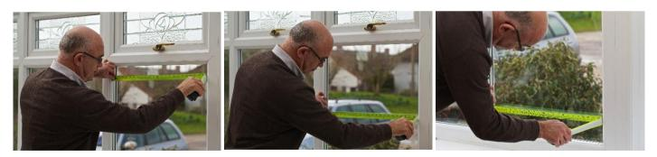
Measure the glass between the bead in 3 places, across the top, middle and bottom. Do the same for the height of the glass. Choose the smallest dimension for both the width and the drop.
