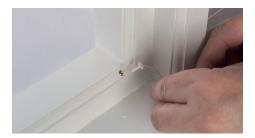
b4. Push knot into brass insert, push grommet into brass insert, aligning groove to cord. (cont. step 11 overleaf).
