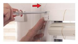
9. Hand screw fixings. (for TF cont. steps b3 & b4 overleaf).
