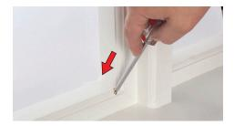
b3. Screw in brass insert until flush with timber surface.
