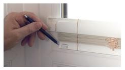
4. Using blind, mark positions for the cord grommet holes. (for TF cont. step b2 overleaf)
