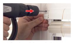
8. Drill two  $\emptyset$ 2.5mm holes on each side.
