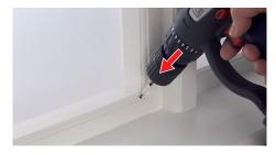
b2. Mark position as outlined in step 4 (overleaf). Drill one Ø4mm hole to a depth of 10mm on both sides. (cont. step 6 overleaf)
